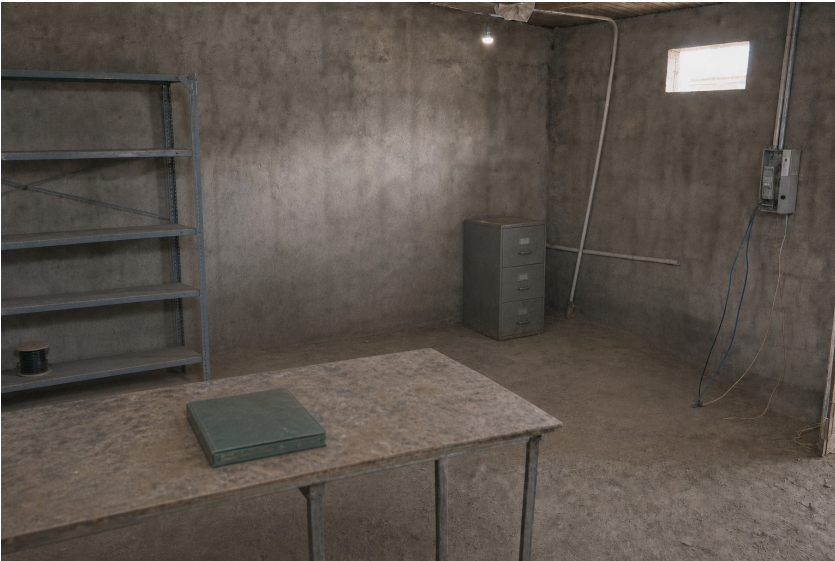
Today's interior after completing the inventory: metal shelf, table, green maintenance folder, map cabinet and control box. Photo: Ana Belén Vargas, 2026.
