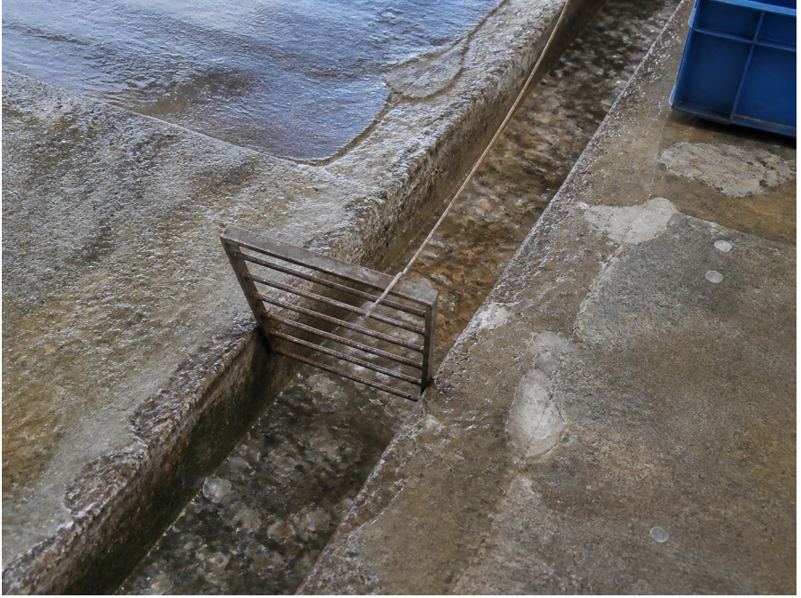
Figure 20. Drainage channel with its cover held open by wire. A simple working solution, photographed in 2026.
