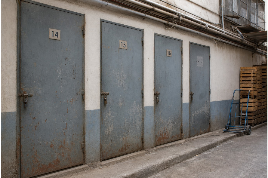
Figure 29. Storage-room doors 14, 15, and 16, and the unlabeled fourth door. Straight-on documentation in neutral daylight, 2026.
