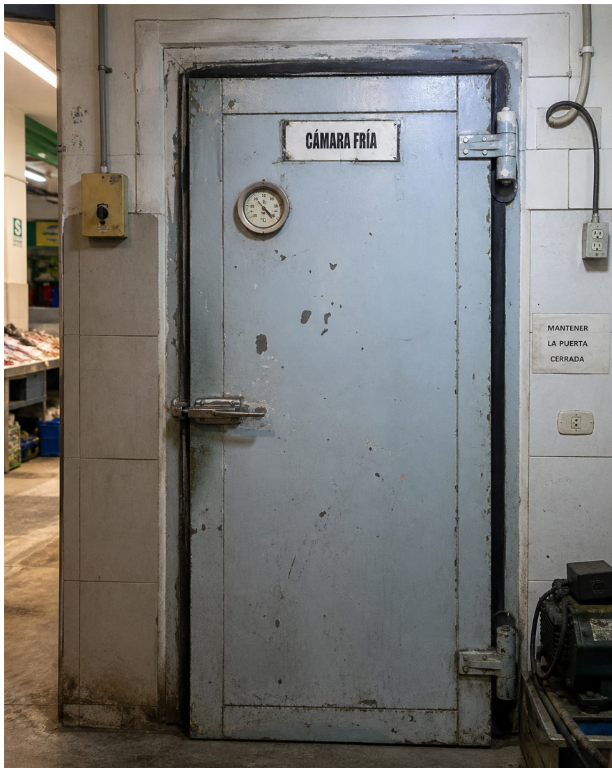
Figure 22. An older cold-room door with a thermometer and numerous traces of repair. No single coat of paint represents the entire period of use.
