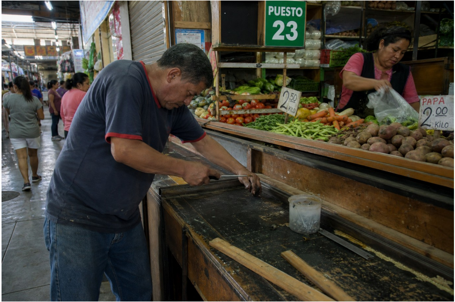
Figure 38. Repairs to a market stall during business hours. Trading continues around the work.
