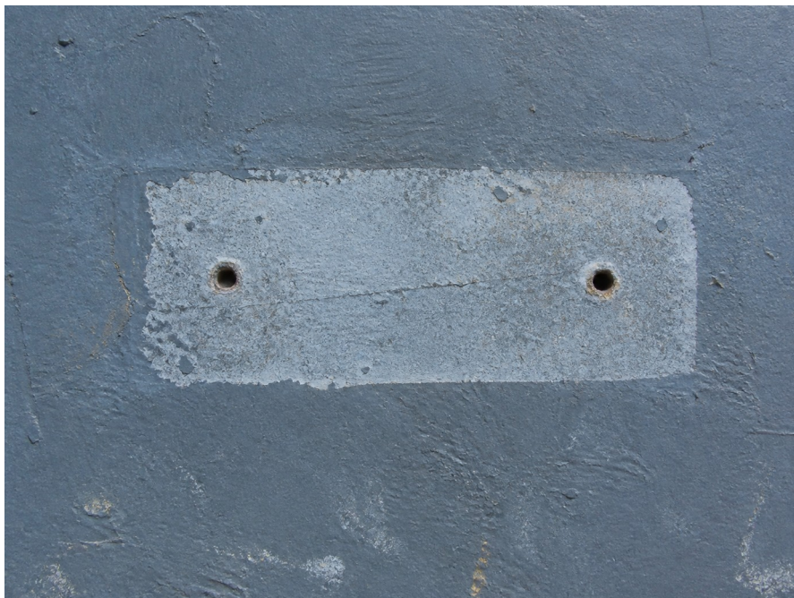
Figure 30. Detail of the missing plaque: a lighter area of paint, two screw holes, and abrasion. The surface evidence does not establish any previous number with certainty.
