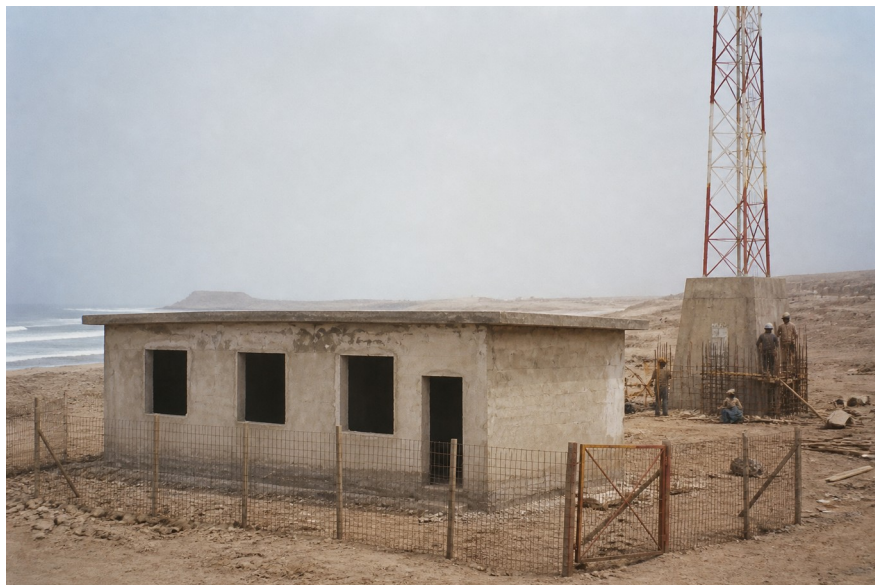
Station building during completion, probably in 1987. The exact date the photograph was taken is not known.
