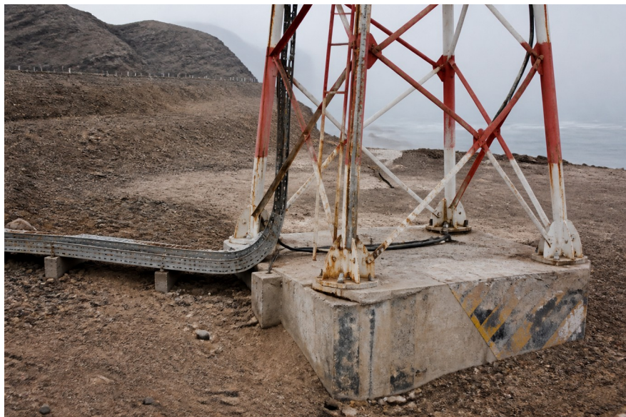
Mast foundation and cable feed. Photograph: Ana Belén Vargas, 2026.
