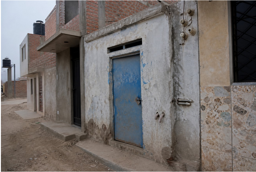
Figure 5 · The older Caseta on Celia Rios's property in Las Palmeras. The residential building was later expanded to include the concrete room.
